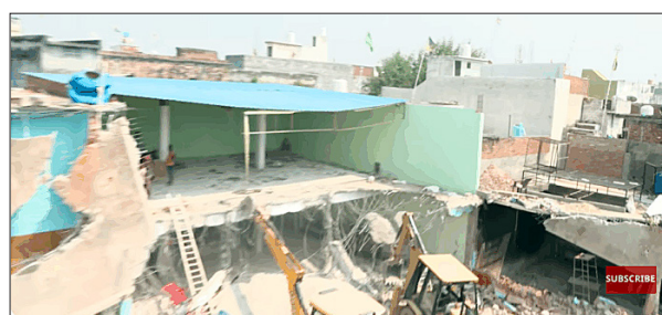
BDA Demolishes Portion of Dr. Nafees's Raza Palace Amid Rising Communal Tensions in Bareilly
