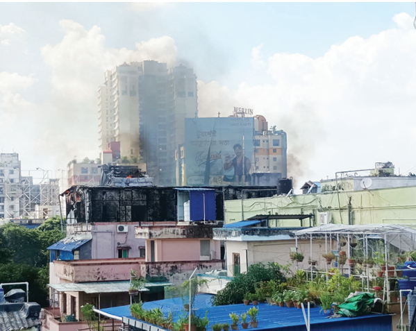
Massive fire at a guest house on Prince Anwar Shah Road in Kolkata on Thursday.
