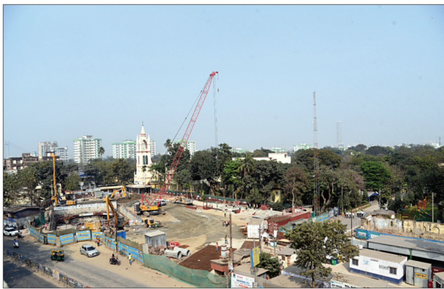
Joka-BBD Bag Metro rail work in progress at Khidderpore, Kolkata.
